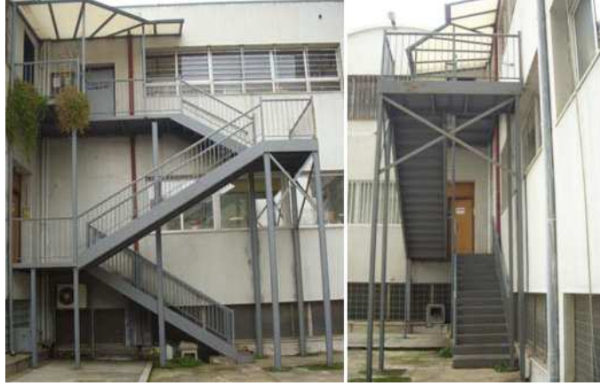
FIGURE 1. The steel stairway in front (left) and side (right) views.
