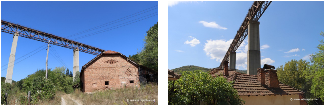
Figure 9. Viaduct Kriveljski Most
