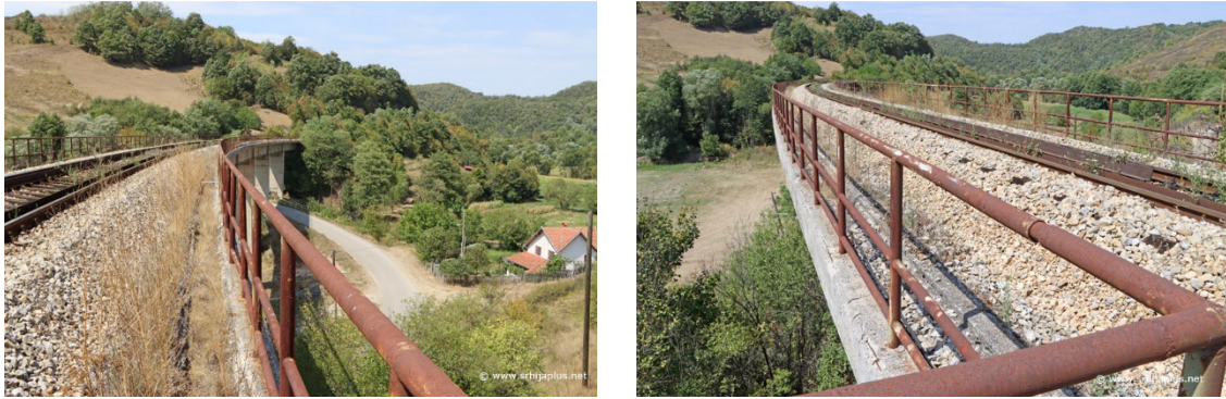
Figure 5. Viaduct Vlaole Selo
