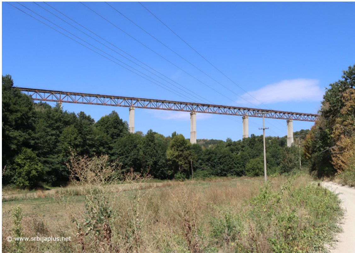
Figure 7. Viaduct Kriveljski Most
