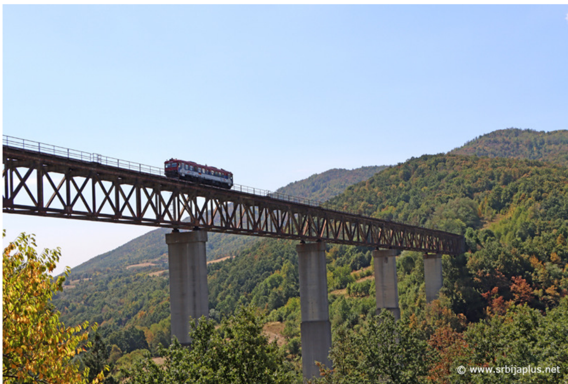
Figure 8. Passenger train crossing the Kriveljski Most
