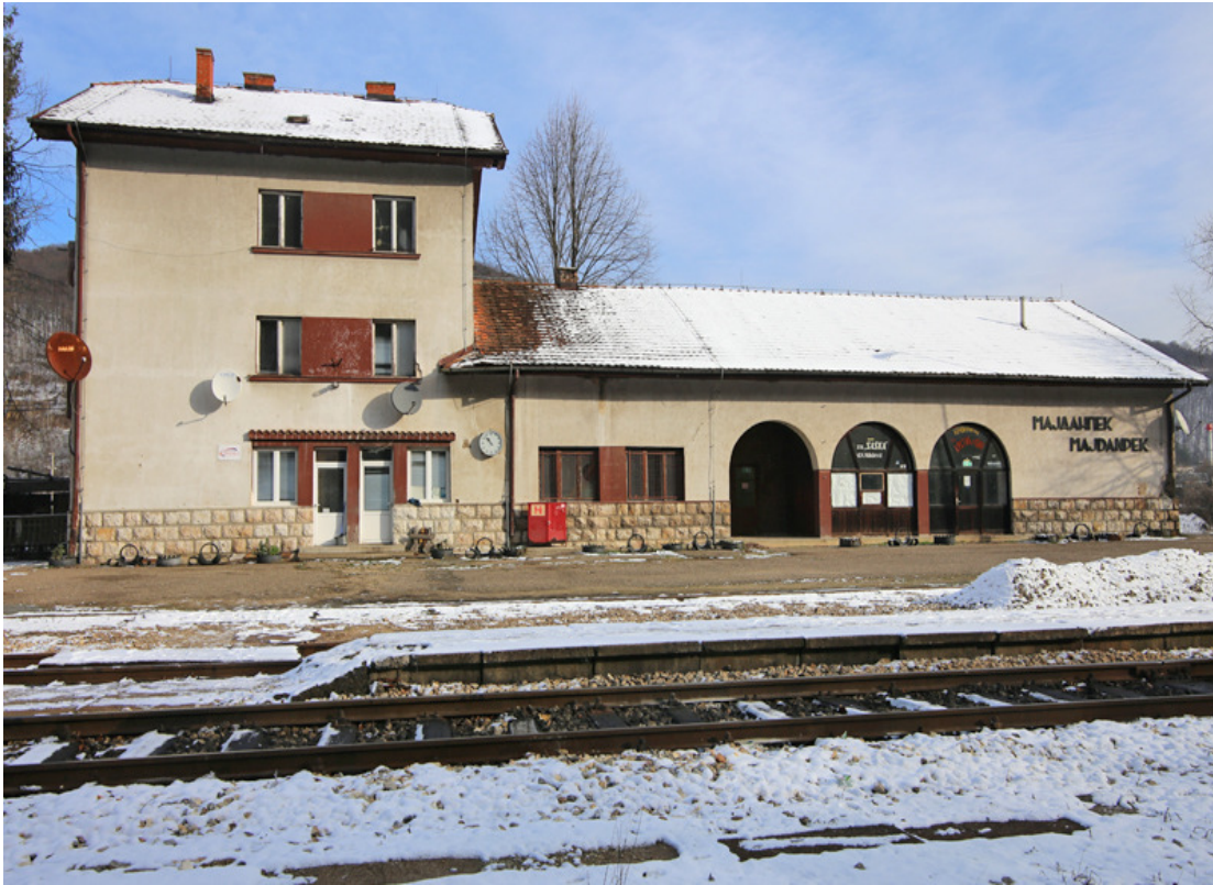
Figure 11. Majdanpek Railway Station
