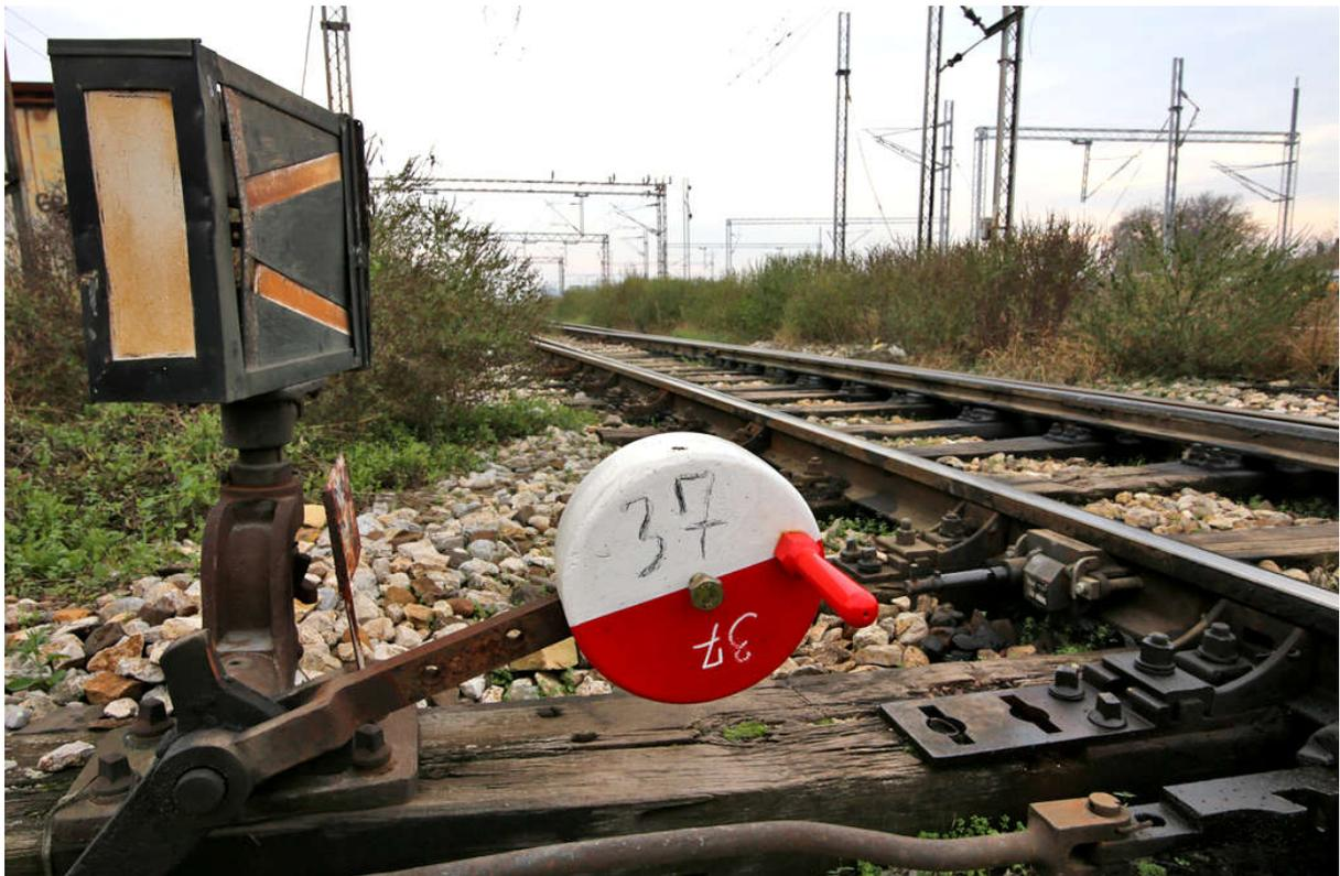
Figure 8. The handrailroad switch, Batajnica, November 3, 2020 (Photo: Z. Cvetković)
