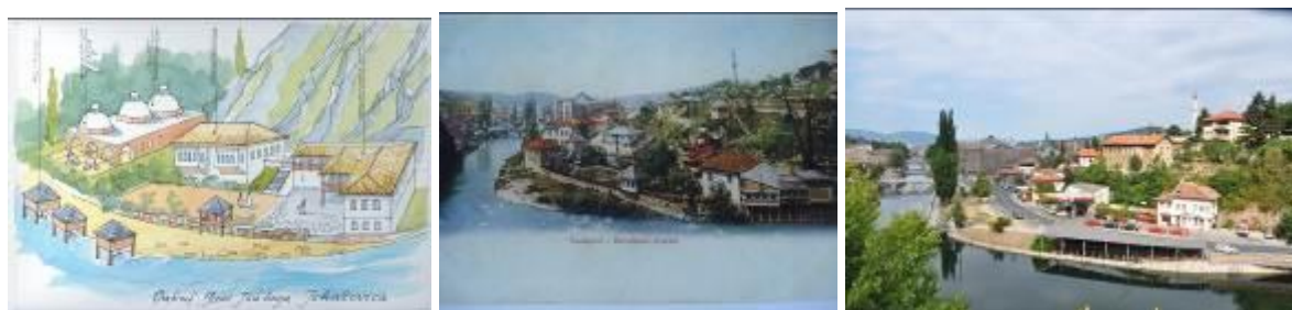
Figure 1: Appearance of the Isa bey's endowment complex through history: a. assumed in 1462; b. 19 th century; c. today
