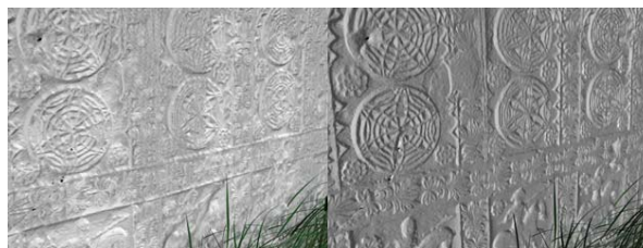
Figure 7: Incorrect orientation (left) and correct orientation (right), 11:00 – close up
