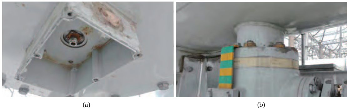
Figure 7: 5062C phase circuit breakers built in sensor
